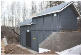
The pre-assembled biomass heating plants are commonly used for municipal heat networks. They are also known as containerized or modular biomass heating plants.
