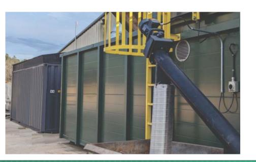
If the moisture content of the available biomass fuel is too high, the hot air generator can be combined with a biomass dryer. The dryer will use a small part of the hot air to dry the fuel before automatically transferring it to the generator.
