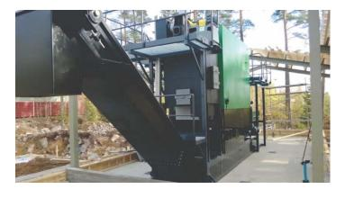
Hot water boilers can be mounted on a skid with most mechanical and electrical installation work done at the factory. This facilitates installation on site and ensures an easy commissioning as the unit is tested before delivery.
